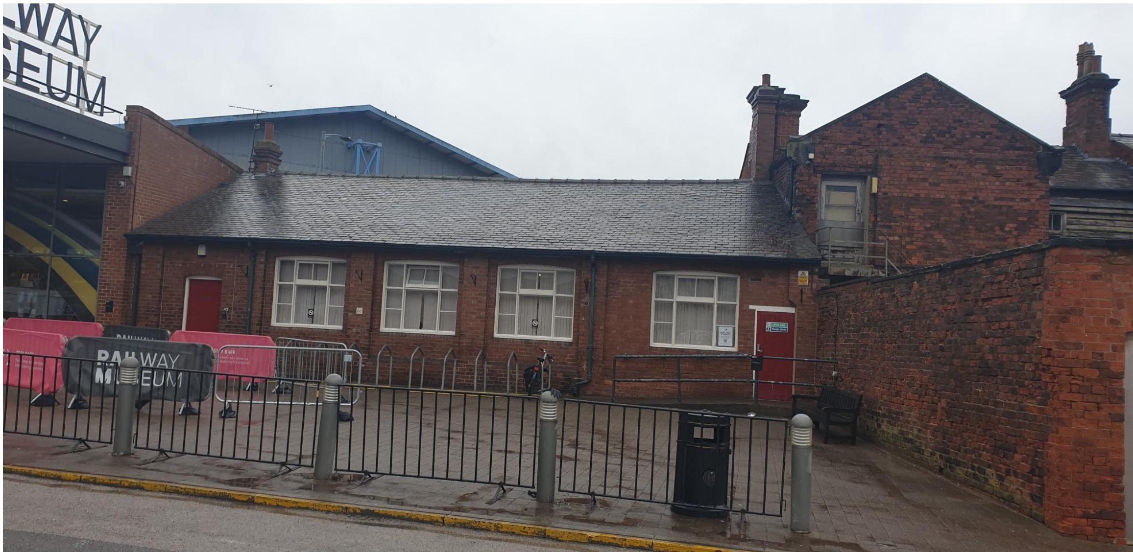
Former mess room to be demolished
